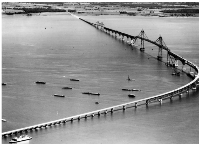
Figure 2: Construction of the Original Bay Bridge Span in 1952
