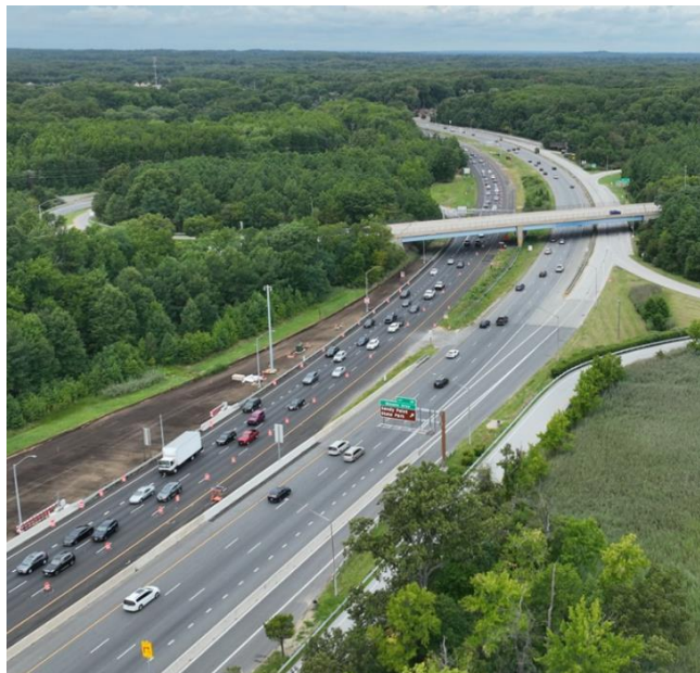
Figure 8: Eastbound queue forming near Oceanic Drive
