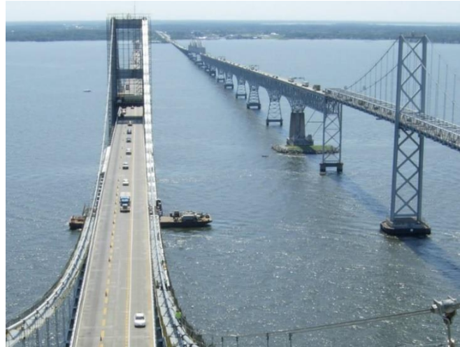
Figure 4: Existing Bay Bridge spans, looking east
