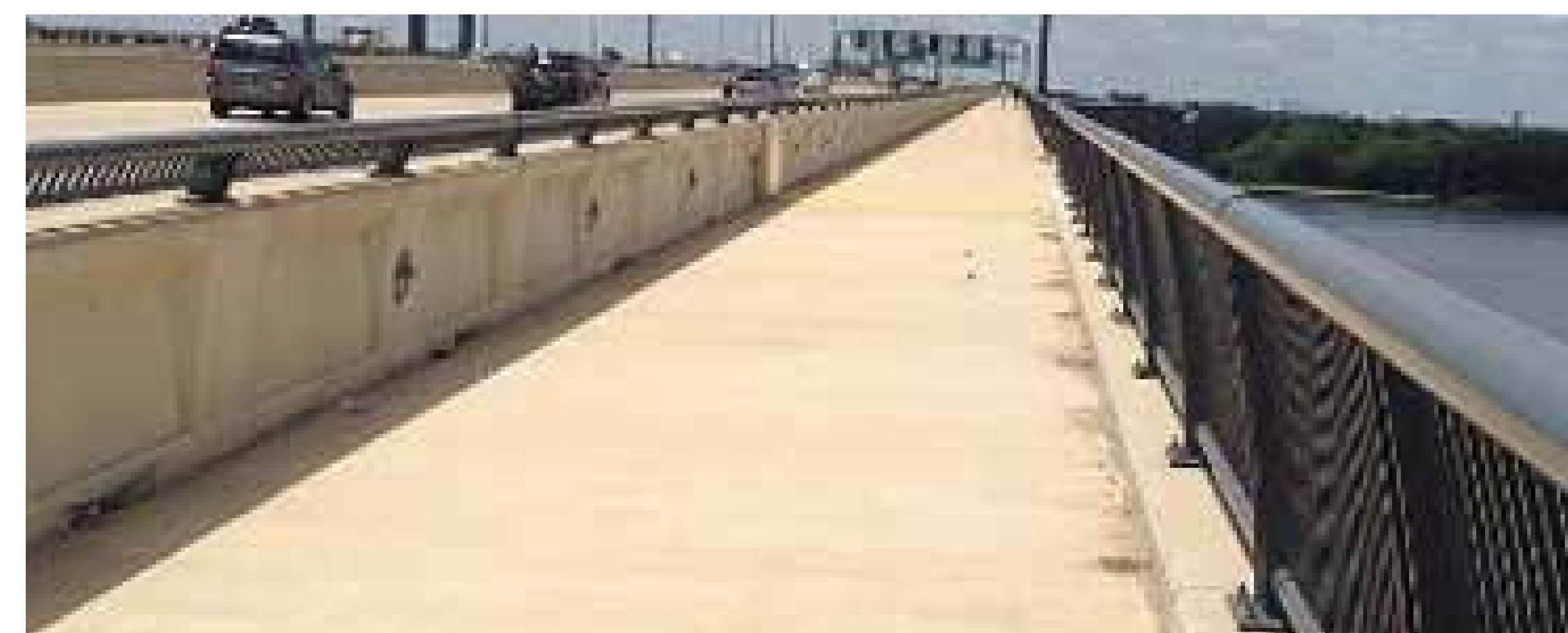
Woodrow Wilson Memorial Bridge (MD)
