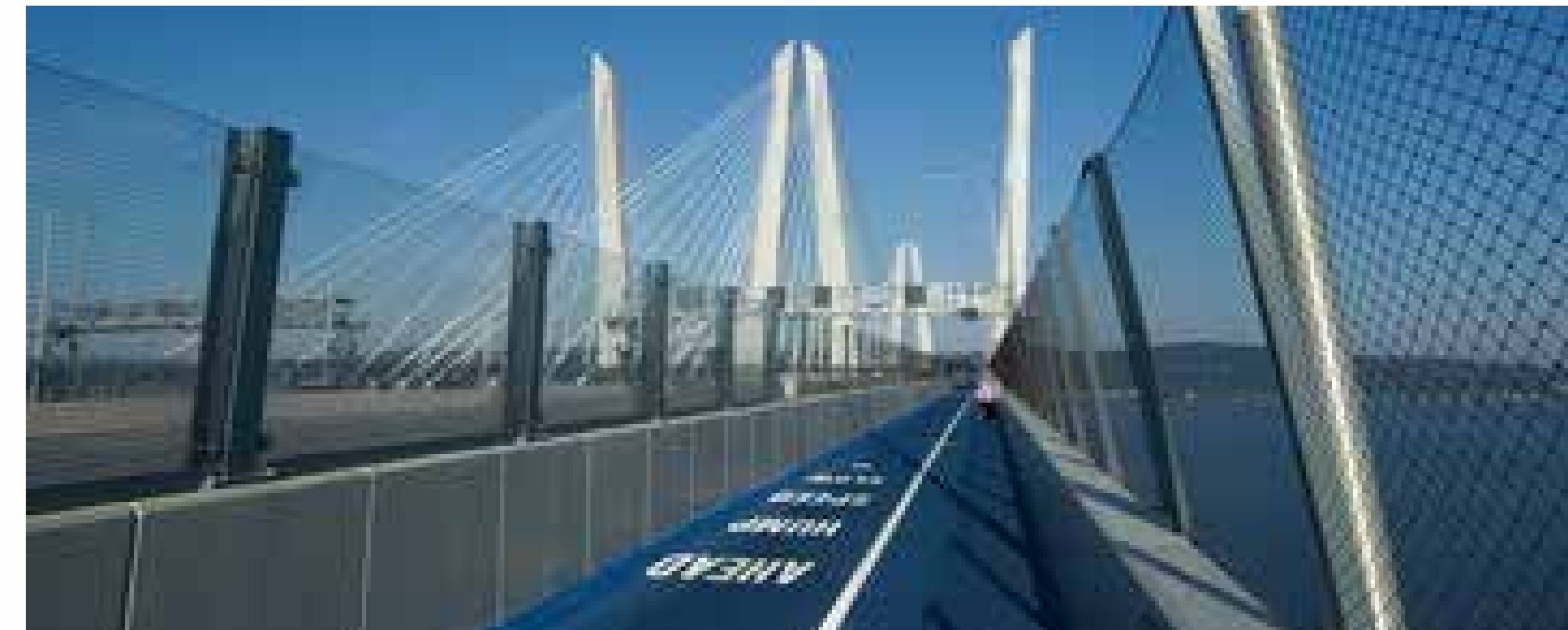
Mario Cuomo (Tappan Zee) Bridge (NY)
