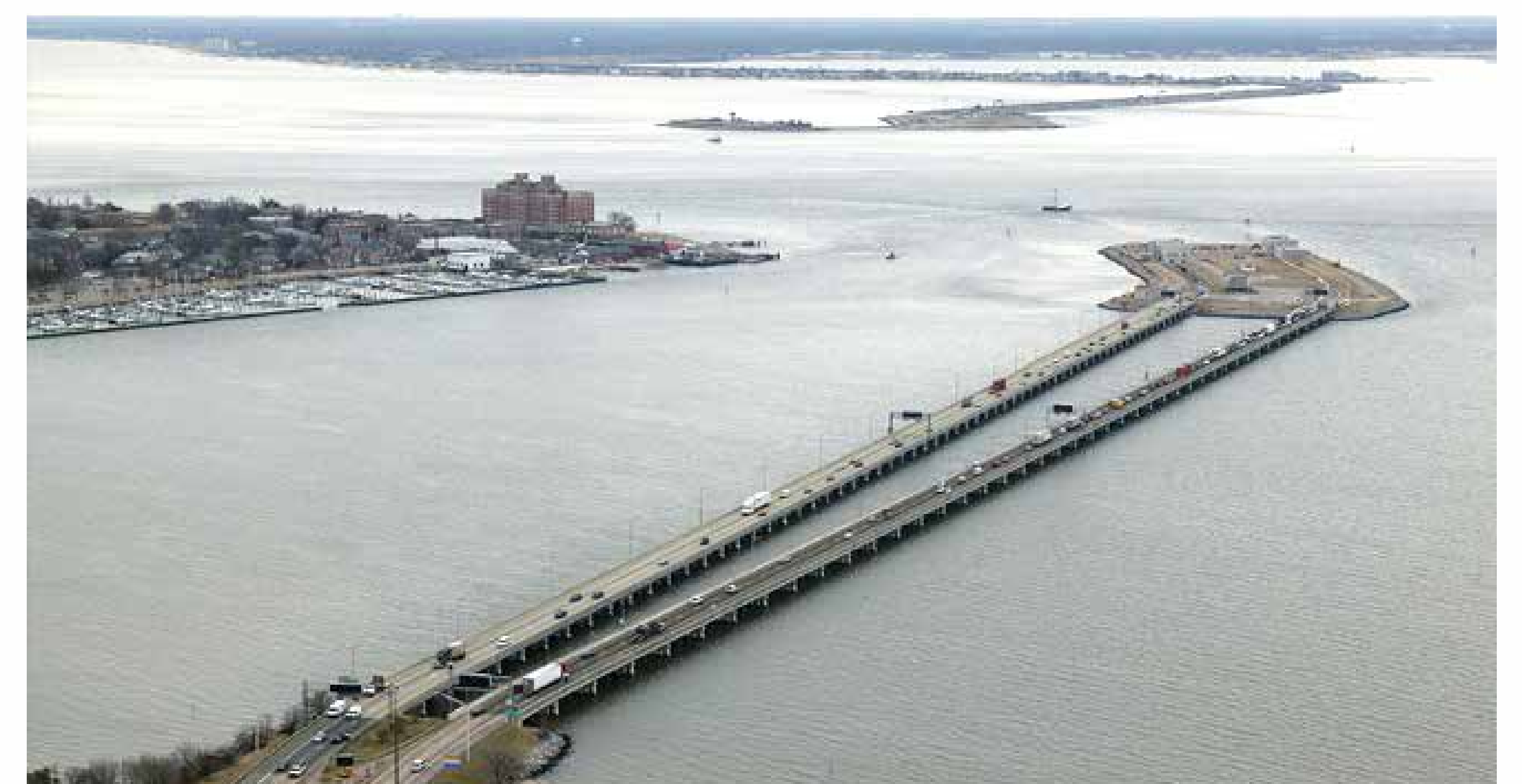
Hampton Roads Bridge Tunnel
